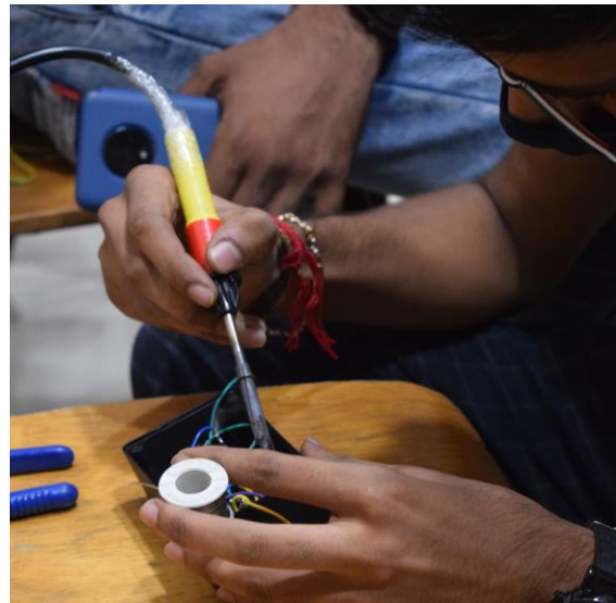
Soldering practice to fix the wire to switch
